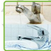
Scaling on Fixtures
